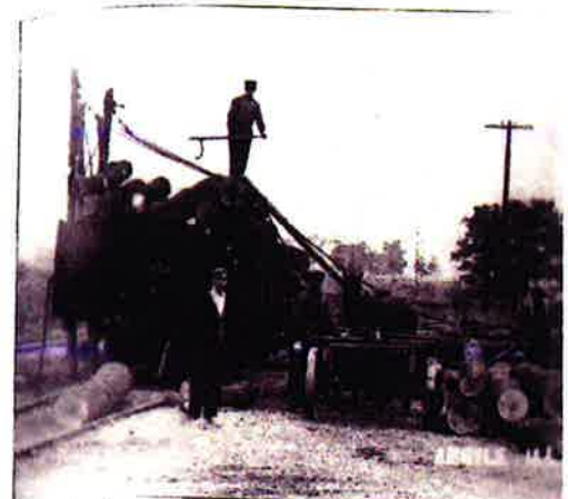
When the photograph was taken early in the 20th century at little A, the rock outcrop 10 miles out of Rockford on Chicago and North line. Workers here, workers take a break from loading fresh cut to go on. In length, a C&NW train will pick up the gondola and to
