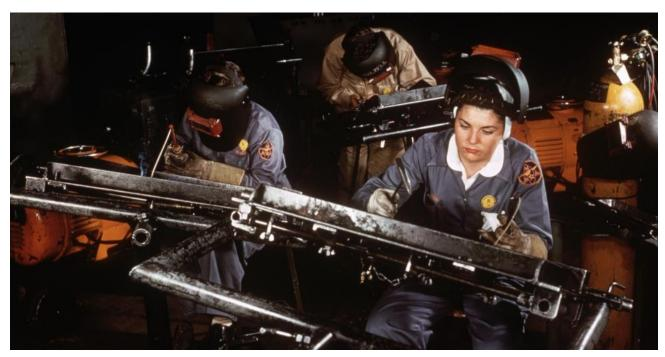
Members of a riveting team at an aircraft factory use rivet guns and bucking bars to work on a basis trainer plane wing center section.
